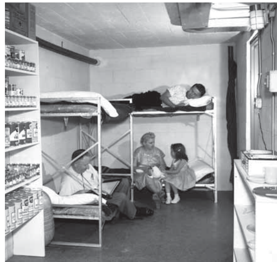
Figure 6. Family Fallout Shelter Residential Interior (U.S. National Archives)
